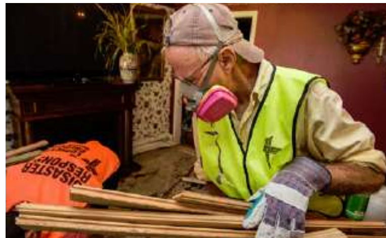
Volunteer Penn Weldon of Thibodaux, La., helps muck-out a flood-damaged home in Baton Rouge, following the August 2016 floods.
